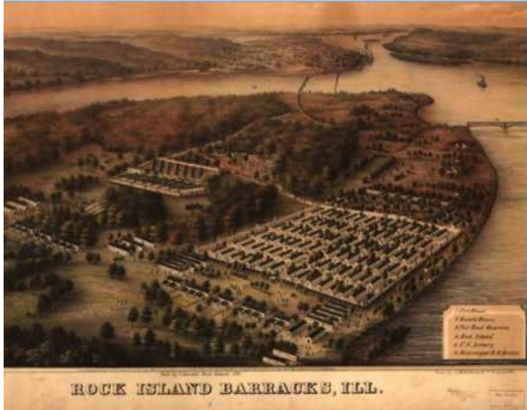
Figure 2.3. The visual order of the city-like prison. This idealized bird’s-eye view depicts the organizational grid that provided order through policing, draining, and ventilating the prison camp at this and other northern prisons. C. Speidal, Rock Island Barracks, 1864, Library of Congress.
